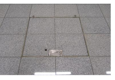
Floor manhole covers are installed to provide access to underground electromechanical network installations (such as air ducts, air conditioning and ventilation systems, fuel or hot water pipelines).
